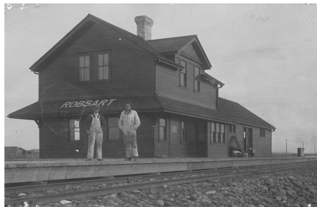
The train station at Robsart, built in 1914. The first station agent was Mr. Sarka.
